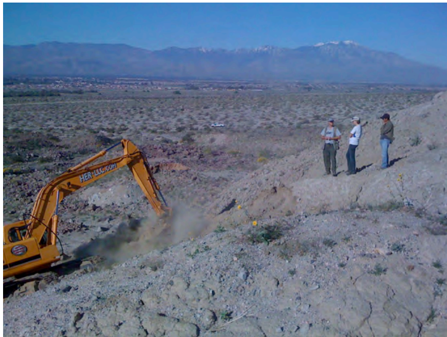
Figure 51. Excavation in progress at Biskra Palms, revealing a relationship at the intersection of the Banning fault with the downstream channel margin. Evidence here is crucial to understanding the long-term slip rate at this site. In addition to re-sampling and dating the T2 surface, numerous excavations were used to test key geological hypotheses related to total offset of the fan surface. Whitney Behr and Nate Guzman discuss new evidence with Prof. Doug Yule (CSUN).
