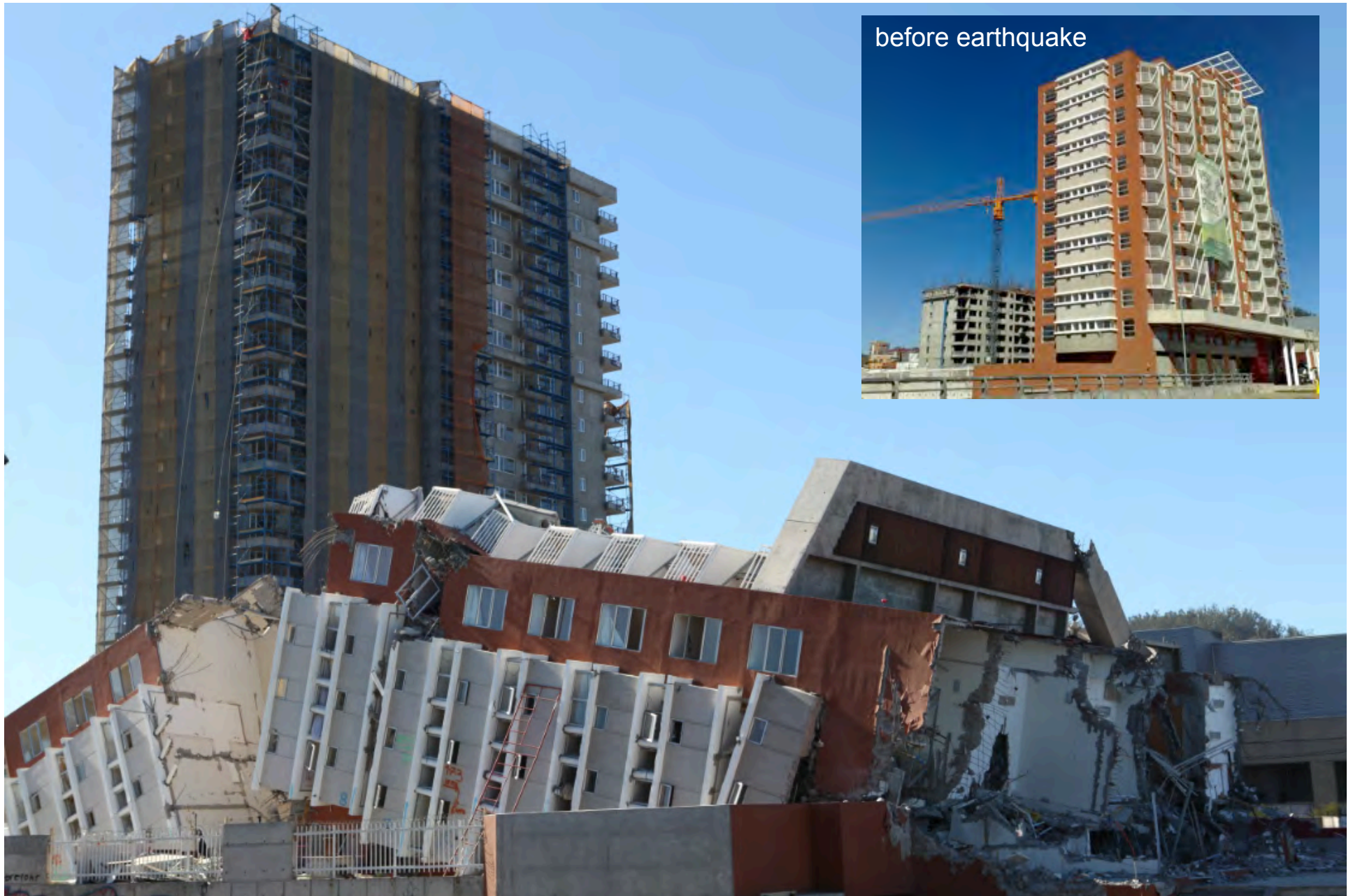
Alto Rio Building, Concepcion, M 8.8 Chile Earthquake Feb. 27, 2010 (Foundation failure)
